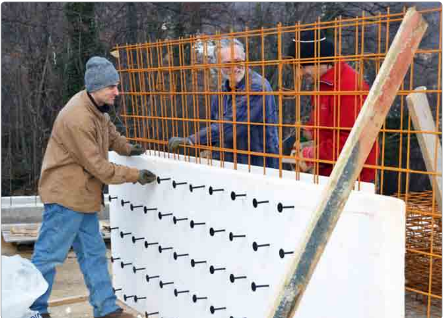
PANEL CONSTRUCTION, WINTER 2011/2012
