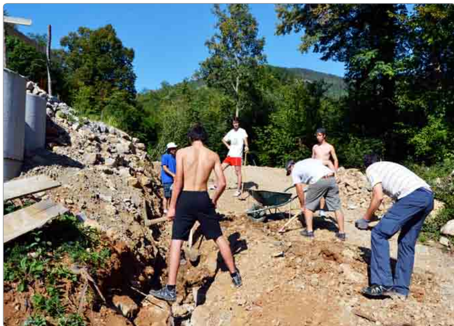
CONSTRUCTION OF THE RETAINING WALL, SUMMER 2011
