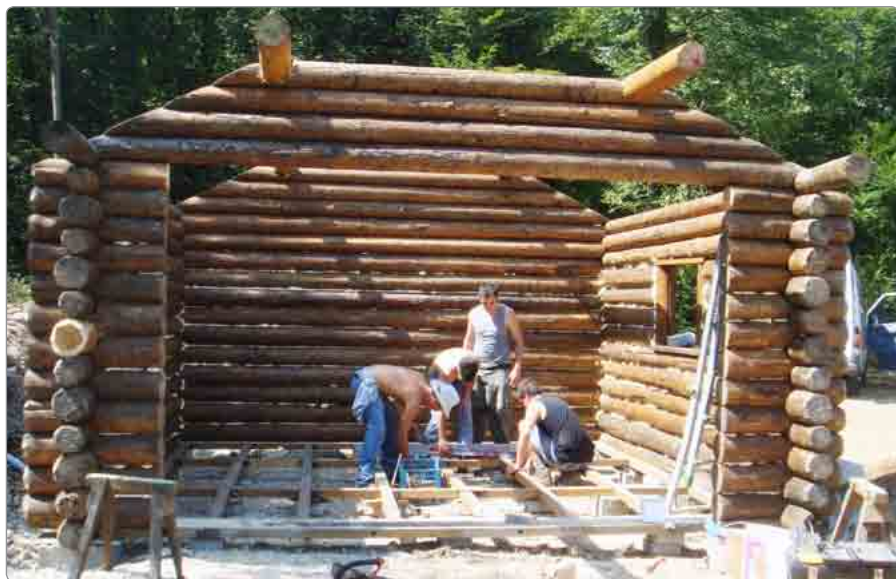
CONSTRUCTION OF THE LOG HOUSE, SUMMER 2010
