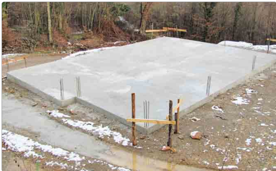
THE FOUNDATION, NOVEMBER 2010
