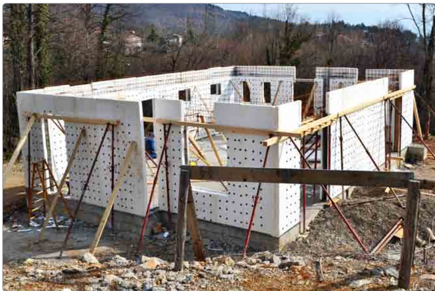
CONSTRUCTION BEGINS, MARCH 2012
