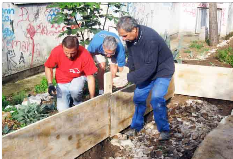
WORK ON DOM ZA ODGOJ, SEPTEMBER 2010
