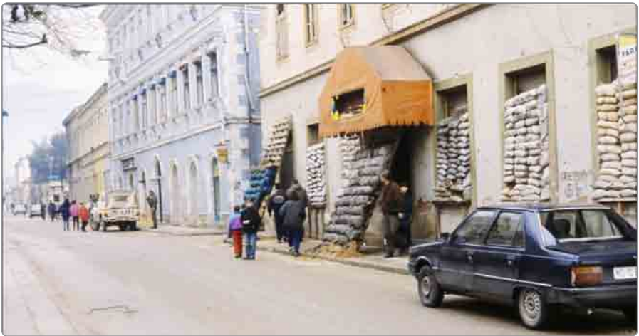
MOSTAR (BOSNIA AND HERZEGOVINA): DOORS AND WINDOWS OF HOMES FORTIFIED AGAINST THE EXPLOSIONS OF SHELLS, JANUARY 1995
